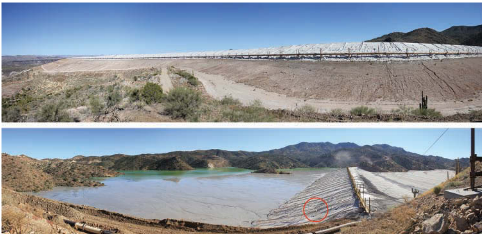
Figure 14-10 View of an Earthen Dam from the Outside (top) and Tailing Pond with an Earthen Dam (bottom)
