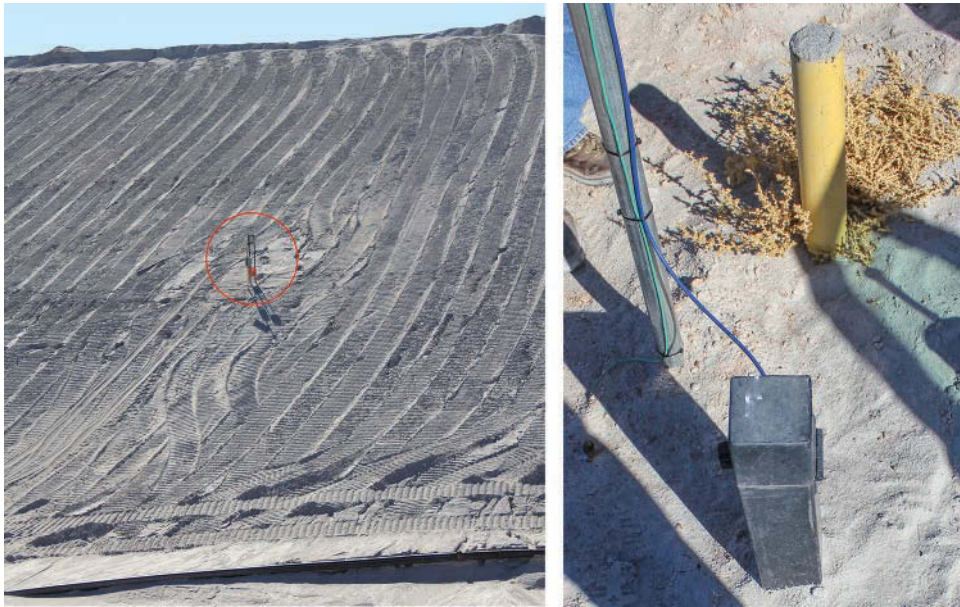
Figure 14-11 A Tailing Pond Earthen Dam with Sensor (Left) and Close-up View of Piezo Ground Monitoring Sensors (Right)
