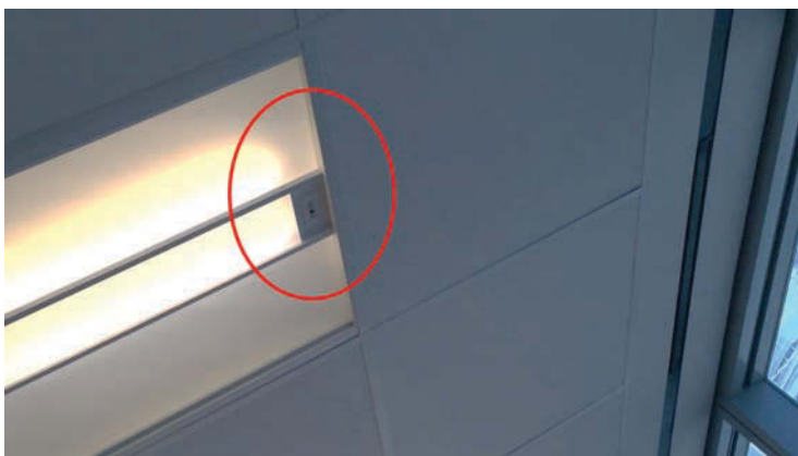
Figure 1-9 An LED Digital Ceiling Light with Occupancy Sensor (Photo by Bill MacGowan)
