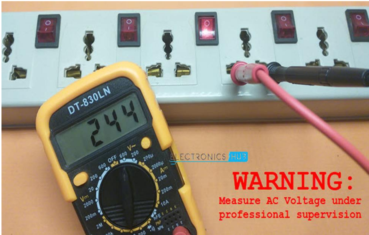
Measuring AC voltage
