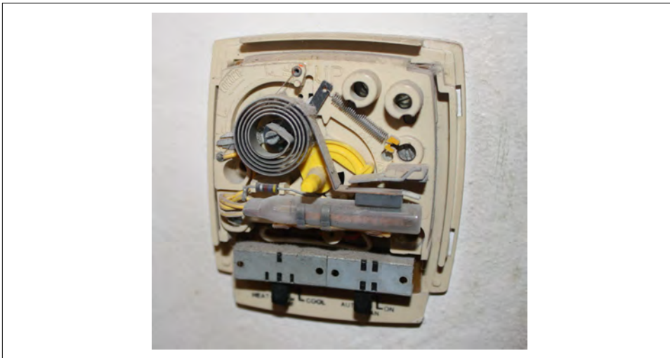
Figure 12-1. Electromechanical thermostat
